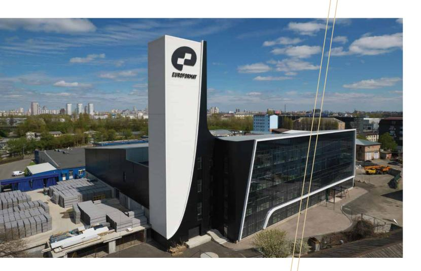
The only elevator test tower in Ukraine operates at the Euroformat new plant. The tower allows testing all of the solutions developed by the plant's design engineers. The height of the test tower is 40 m.
